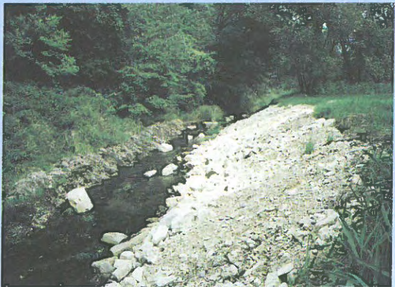
Streambank stabilization (above) is used to prevent erosion. Project Coordinator Frank Moore (below right) works with producer Alan Schatz on integrated crop management.
