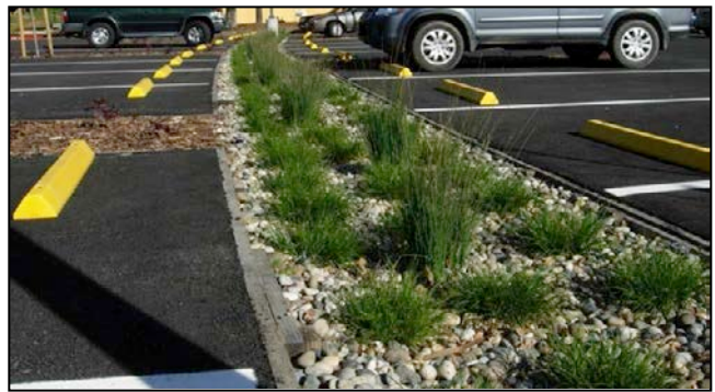
Figure 33 Image of a bioswale adjacent to a roadway to infiltrate the stormwater runoff.
