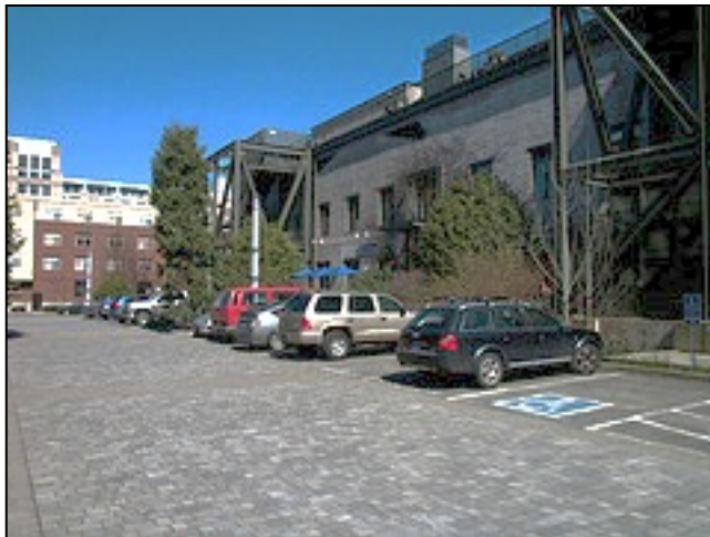
Figure 38 Permeable paver parking lot.
