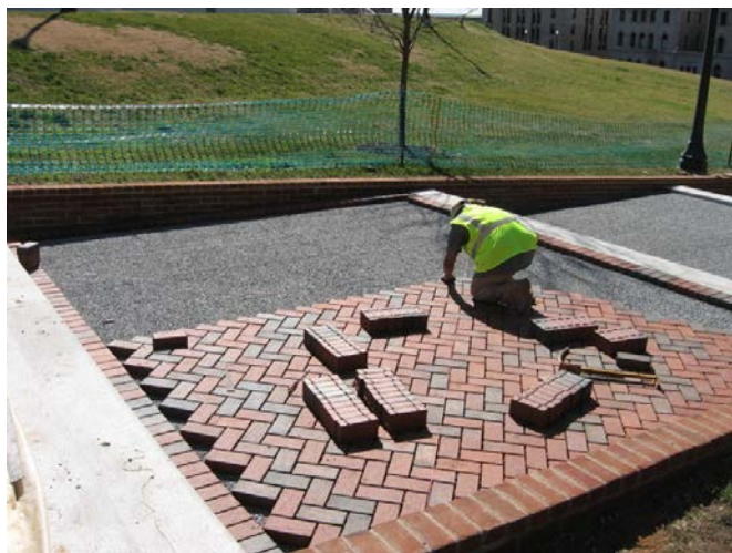
Figure 32 : Permeable pavement system
