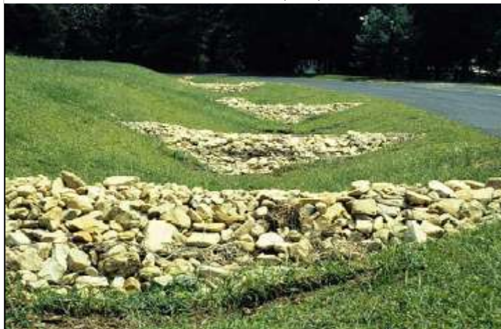
Figure 27 Picture of dam checks alongside a road. This slows stormwater runoff in order to maximize infiltration capacity.
