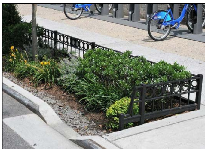
Figure 30 Curb cut-ins direct the stormwater flow into the bioretention cell for infiltration before being directed into the storm drain located sub-surface.
