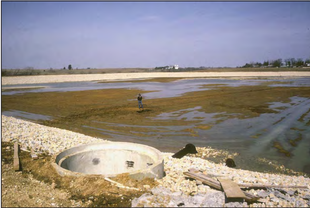
Figure 12-3. City of Garnavillo lagoon after sinkhole failure.
